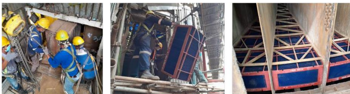
Figure 7. Implementation of a new element of air preheater
