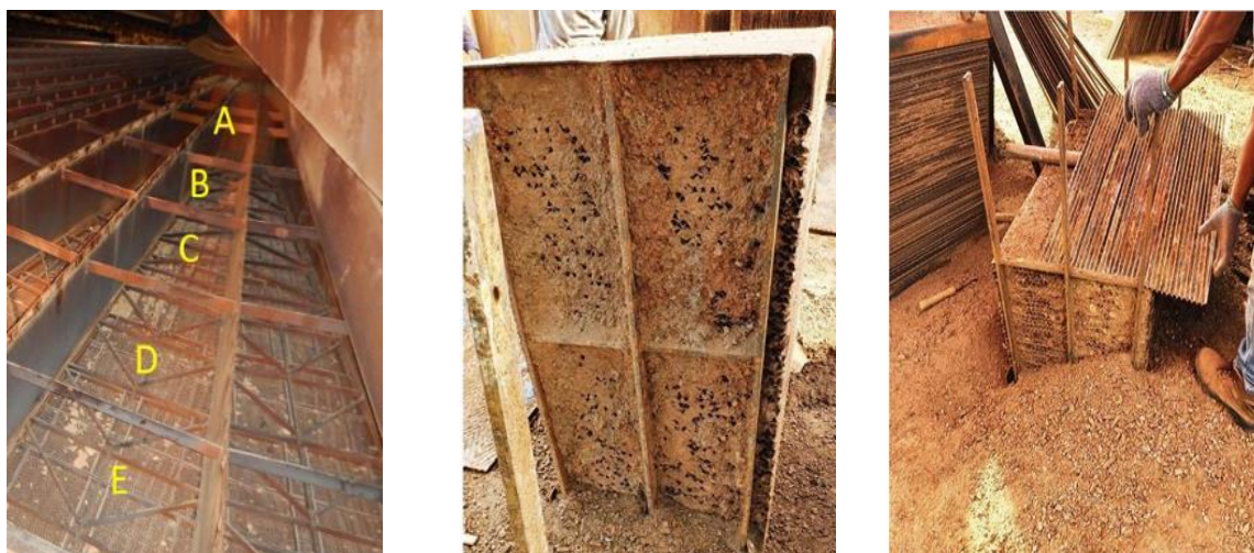
Figure 6. Ash particles carry over to air preheater
