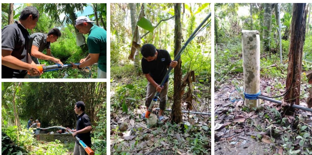
Figure 6. Installation of the Submersible Pump in the Well
