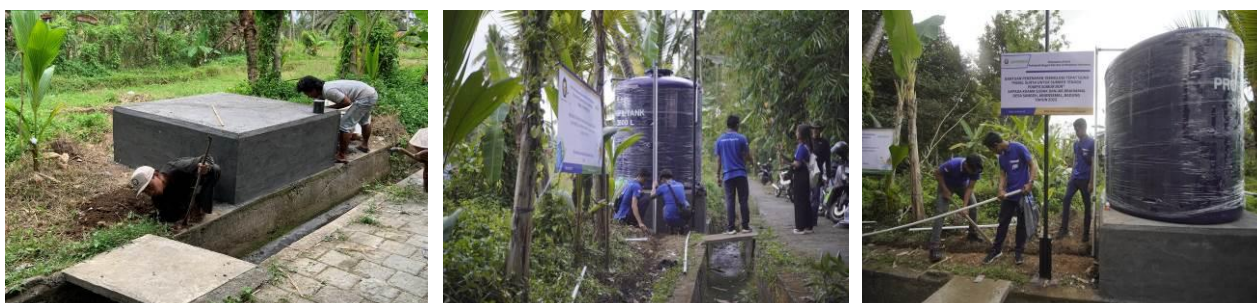
Figure 8. Installation of Water Tank and its Pipes
