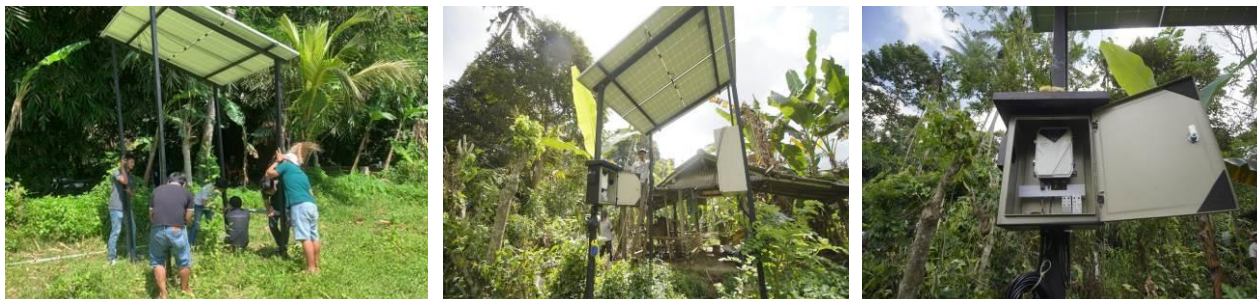
Figure 7. Installation of Solar Panel and Pump Controller
